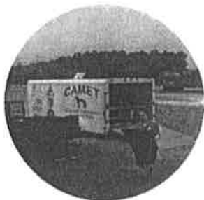
Trailer arrives at site
